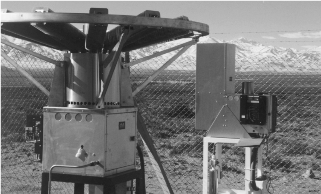
Figure 10.5 Installation of a thermoelectric generator. (Courtesy of Global Thermo-electric, Inc.)
